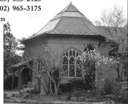
Slate Roof and Gutters replaced in 2004
