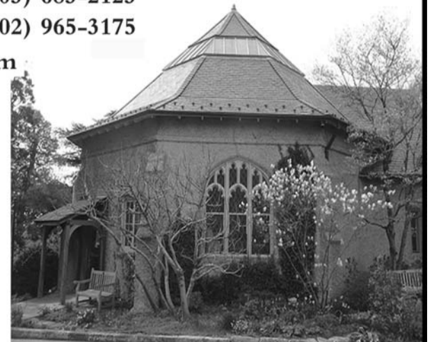
Slate Roof and Gutters replaced in 2004
